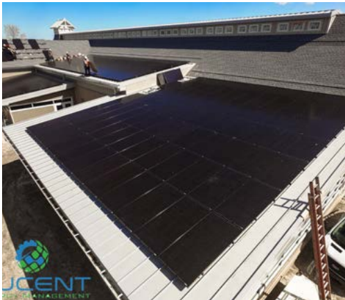
Solar panels on Lewes Library.
